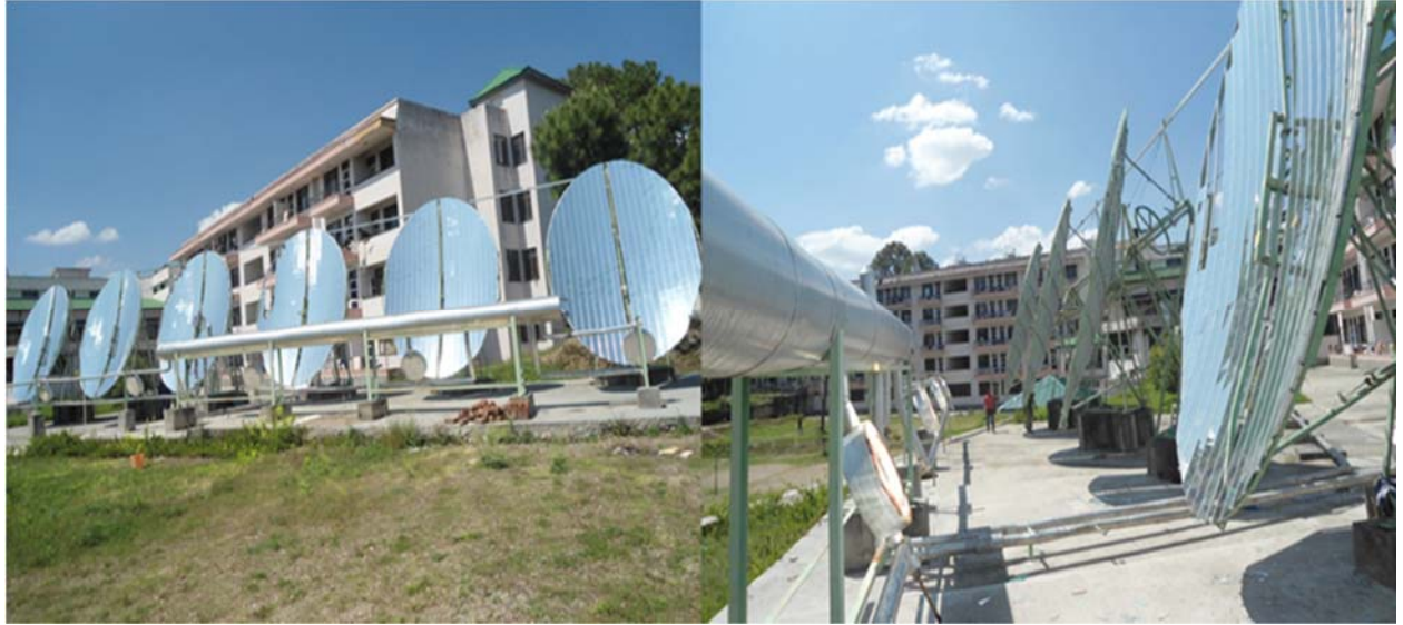
Steam generating cooking system installed at Neelkanth Hostel
